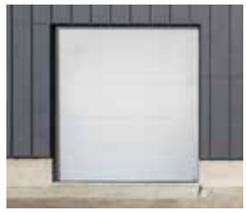
REPAIRED DOOR WITH AMARR 2747 REPLACEMENT SECTION
